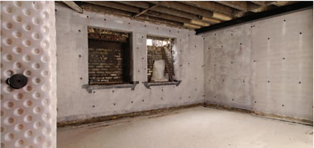
**CM Plaster (or CM8/CM20 with Dab Collars):** use a board adhesive or bonding plaster/adhesive recommended by the board manufacturer in a conventional ‘dot and dab’ application. Ensure at least 50% of the membrane surface area is covered by plaster adhesive and to a final depth of 8 mm. Provide
