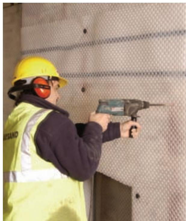
Step 1: Drilling through the membrane to accept fixing plug.
