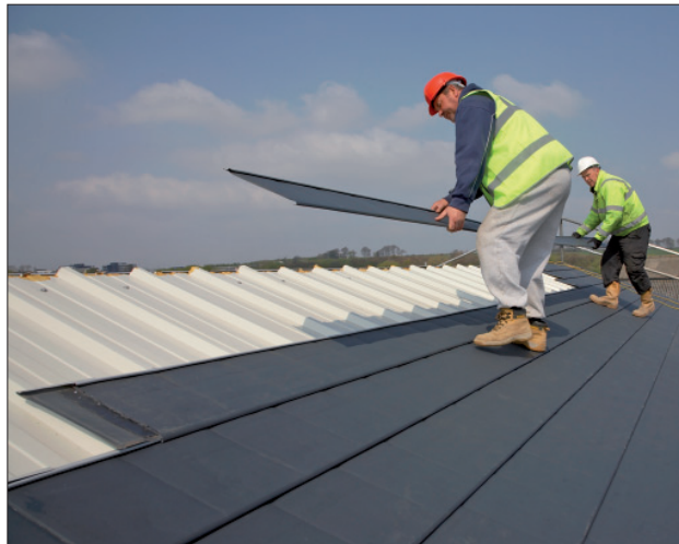
Figure 5 View of Meta-Slate Plus being installed
