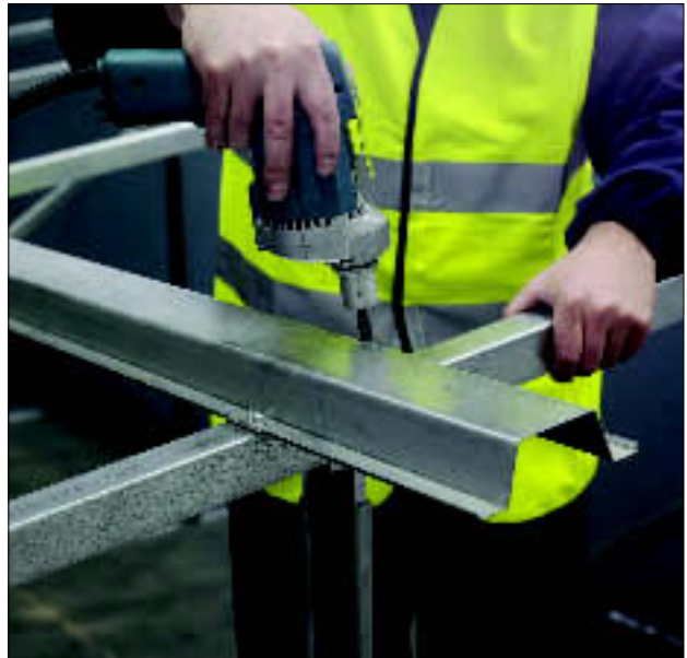
Figure 7 Purlin fixed to rafter
