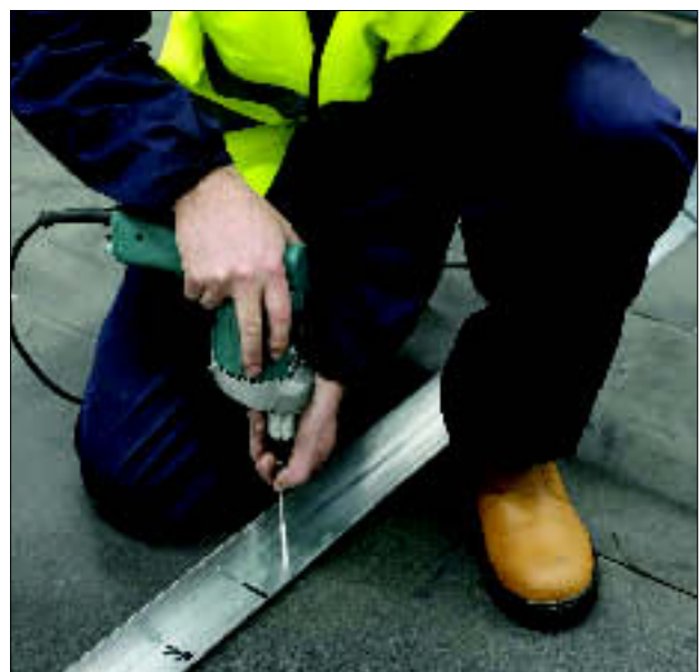
Figure 3 Base spreader fixed into position
