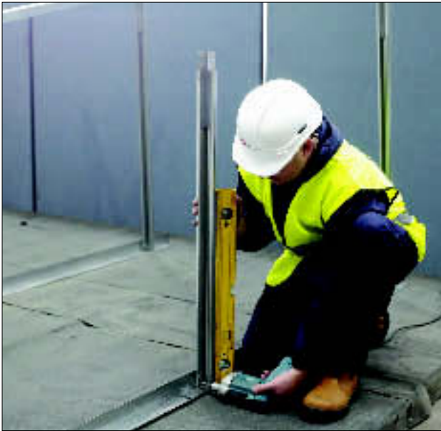
Figure 5 Base fixed to prop
