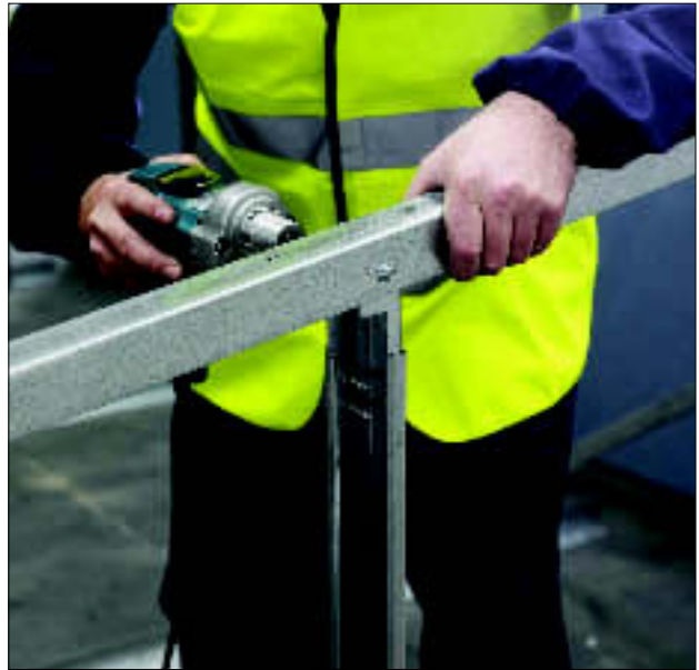
Figure 7 Purlin fixed to rafter
