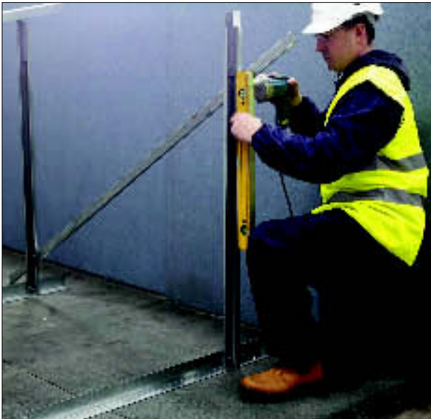
Figure 5 Base fixed to prop
