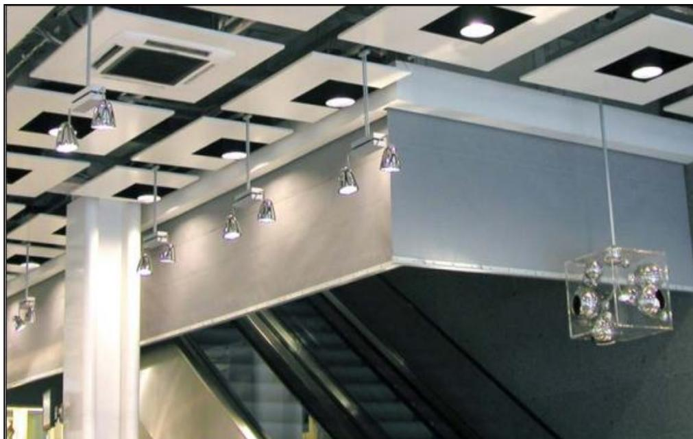
Smoke curtains can be supplied in unlimited widths by use of our overlap system with curtains up to 5 metres wide being serviced by single span rollers.
