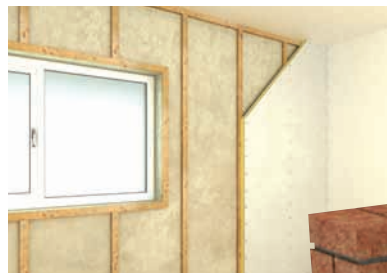
Thermal Liner DOT & DAB - Typical installation
