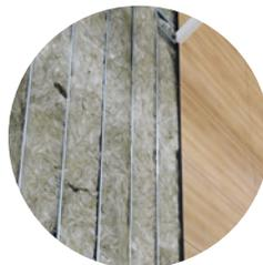
Insulation must be placed behind the panels to achieve required thermal and acoustic values.
