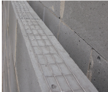
Bed-joint reinforcement
