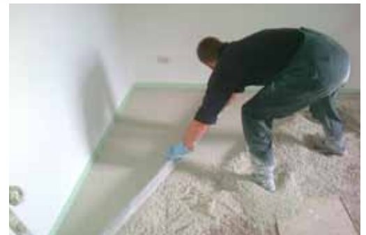
GEOCELL foam glass bubbles: bound fill
