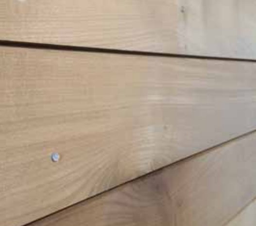
Brimstone® Sycamore cladding
