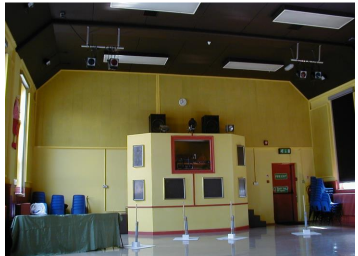
Internal Application of Siderise WPM System with Polyester Powder Coated panels & cover strips
