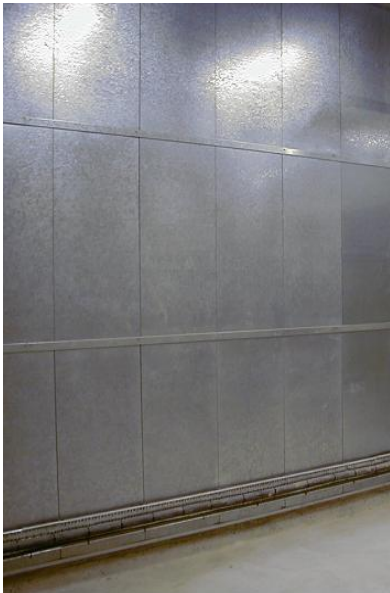
Internal Application of Siderise WPM System on Walls and Ceiling
