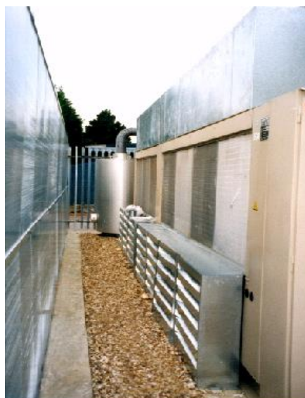
External Application of Siderise WPM System
