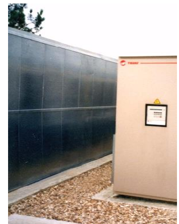
External Application of Siderise WPM System
