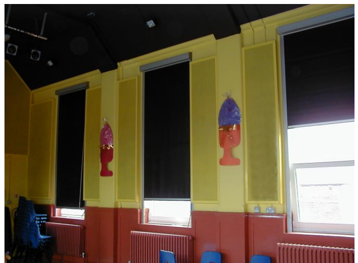
Internal Application of Siderise WPM System with Polyester Powder Coated panels & cover strips
