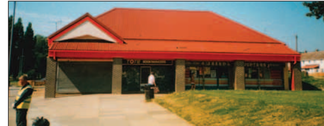
Boldroll ridge to eaves tile effect roofing sheets offer improved structural integrity over traditional materials, making them a popular choice for areas with high levels of vandalism.
