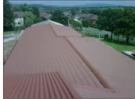
The Boldroll ridge to eaves roofing system can be used on projects where the weight of traditional materials is too great.
