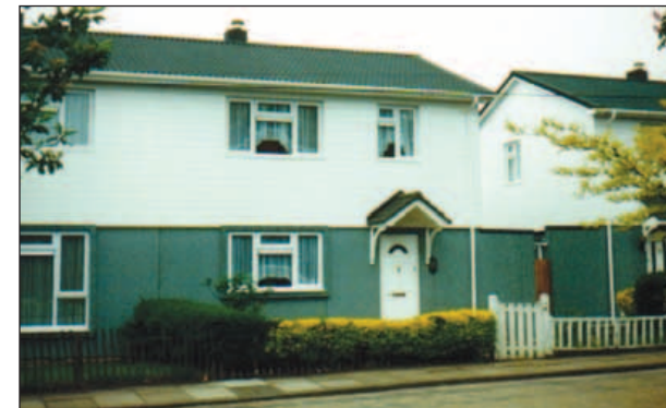
The Pantile 2000 fast-track roofing system considerably reduces time on site, keeping disturbance to a minimum.
