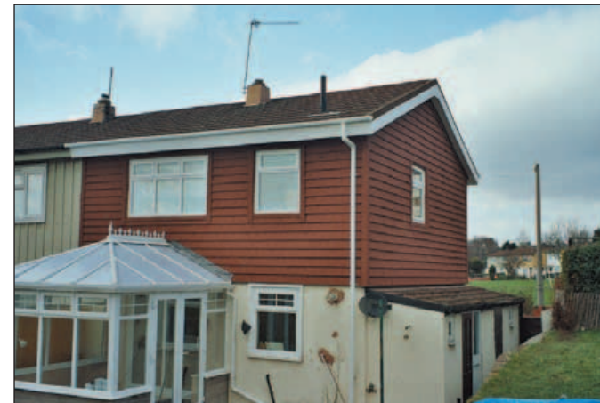
The Plain Tile's aesthetic characteristics permit its use in a wide variety of applications including vertical cladding.
