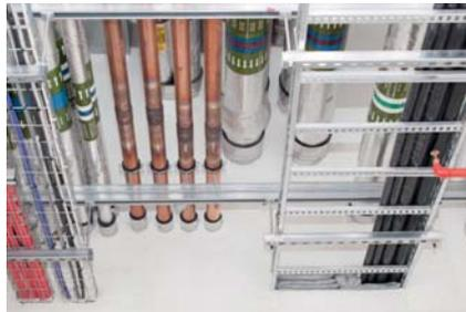
All service penetrations will allow for various combinations of plastic and metallic pipes, ducts, power and data cables. Each element will react very differently to fire, this requires that the fire stopping systems are designed, manufactured and installed to cope with the individual needs of the project.
