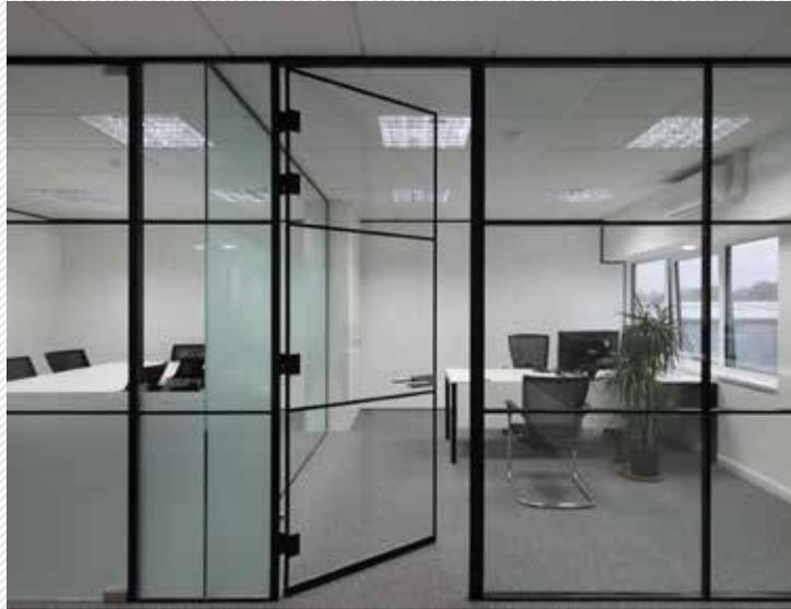
Based upon framing of just 16mm thick, IsoTec's 12mm toughened glass door leaf is surrounded by aluminium. Either match or contrast with the corresponding partitioning's framework by polyester powder coating it in a vast range of colours or anodised, for a metallic finish. Glass with protected glass edges is a benefit as the framing prevents glass to glass edges from damage.
