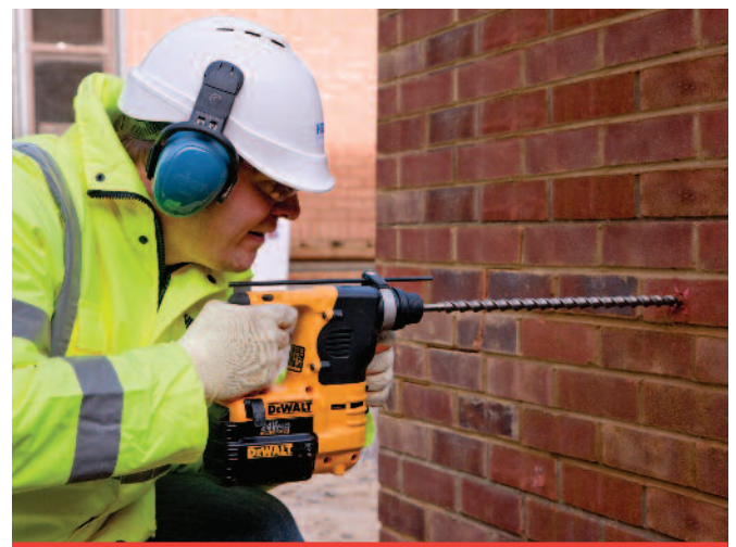
Drilling clearance hole in both leaves ready for CemenTie installation
