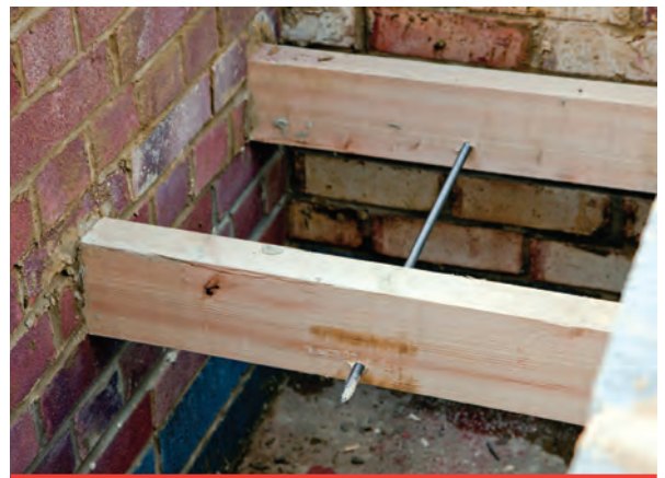
BowTie HDs installed through parallel floor joists
