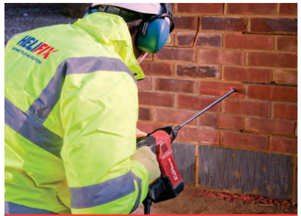
Drilling clearance hole for installing BowTie into joist end
