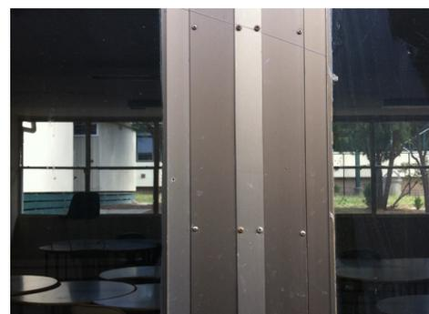
It is a difficult art when anodizing light and heavy parts to achieve the same depth of color, as heavy parts require longer in the tank and the final color is not apparent until after the anodizing is complete.
