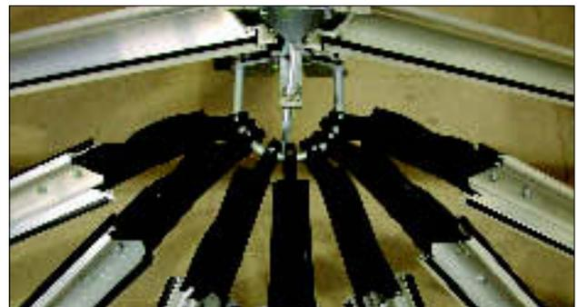
1.7 Glazing panels or units supported by the glazing bars are located into the ridge system through a PVC-U glazing trim with a TPE co-extruded gasket, which provides a seal against the
