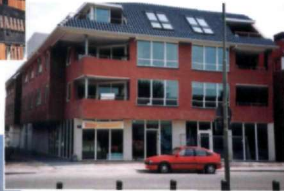
Balconies and overhangs
