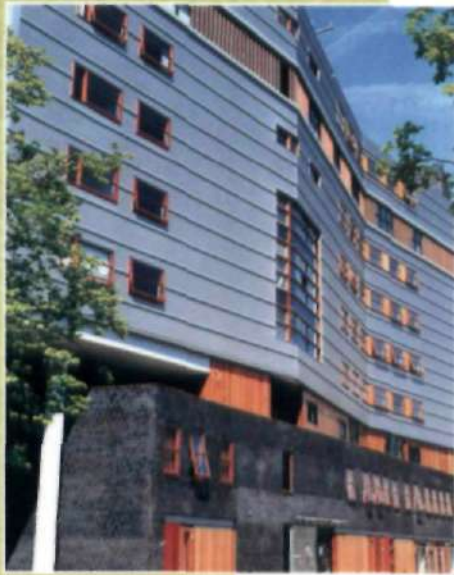
Ground Floor parking in domestic buildings
