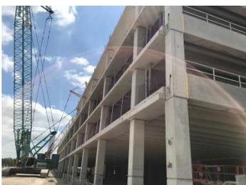
Utilising precast concrete beams and columns is an aesthetic and efficient method of concrete frame construction. Increasingly, architects seek visibility of the structural form, whilst maintaining elegance and structural integrity.
