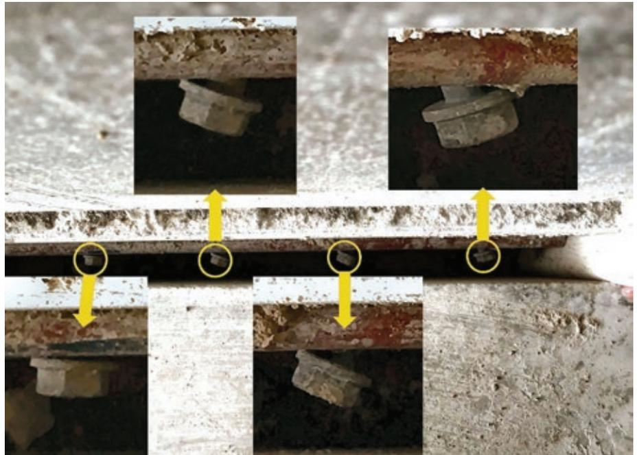
Figure 1: Badly seated fixings due to hitting steel.
