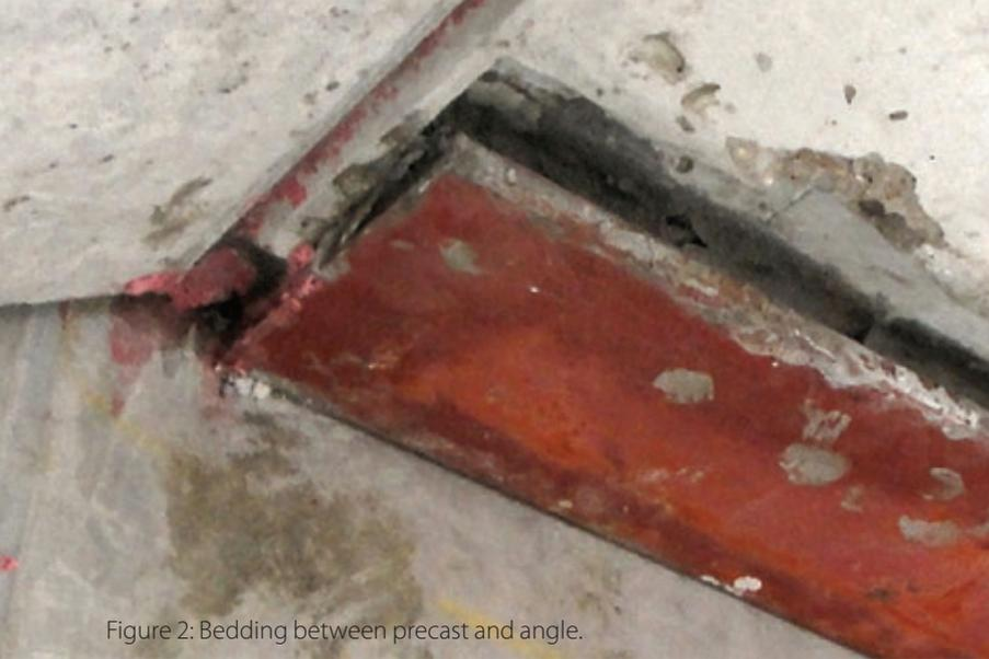
Figure 2: Bedding between precast and angle.
