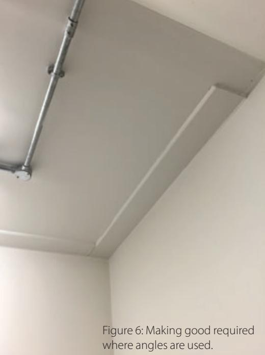
Figure 6: Making good required where angles are used.
