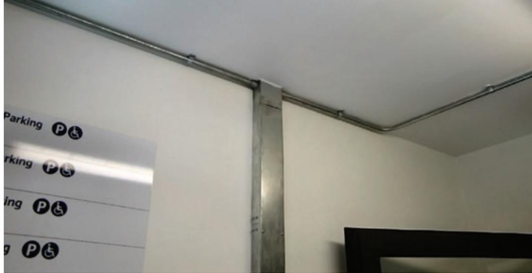
Figure 7: Clean soffit achieved with telescopic connectors.
