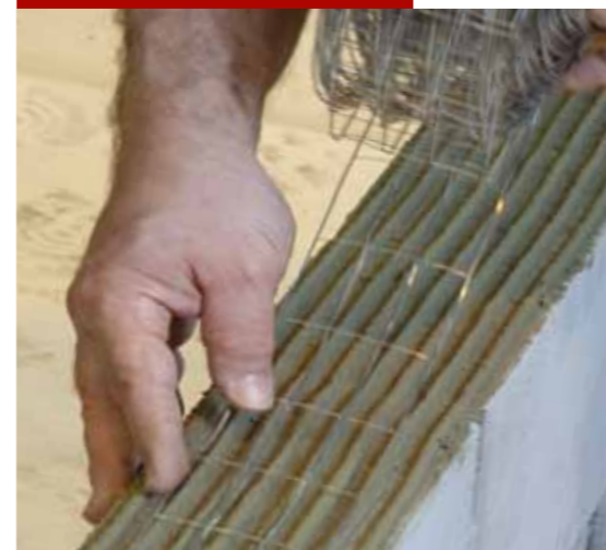
2-3mm Thin Joint System
