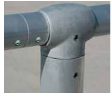
mechanical fixings to all connections
