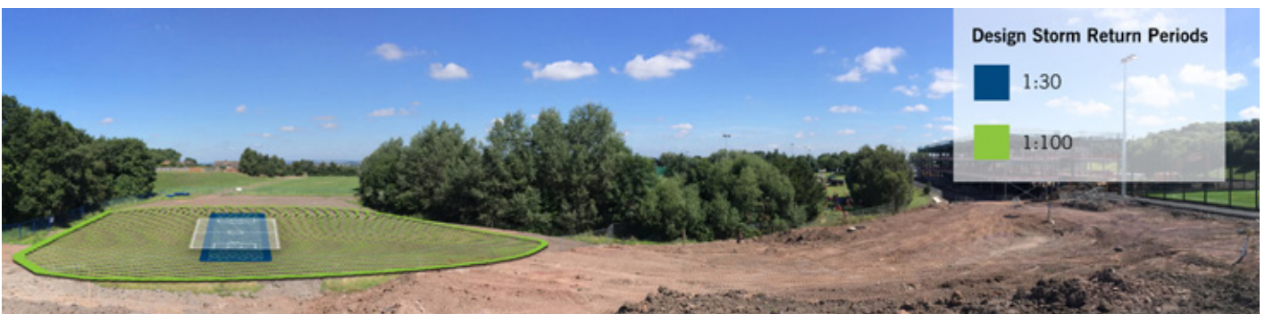
Graphic highlights the attenuation capacities of this SuDS design.
