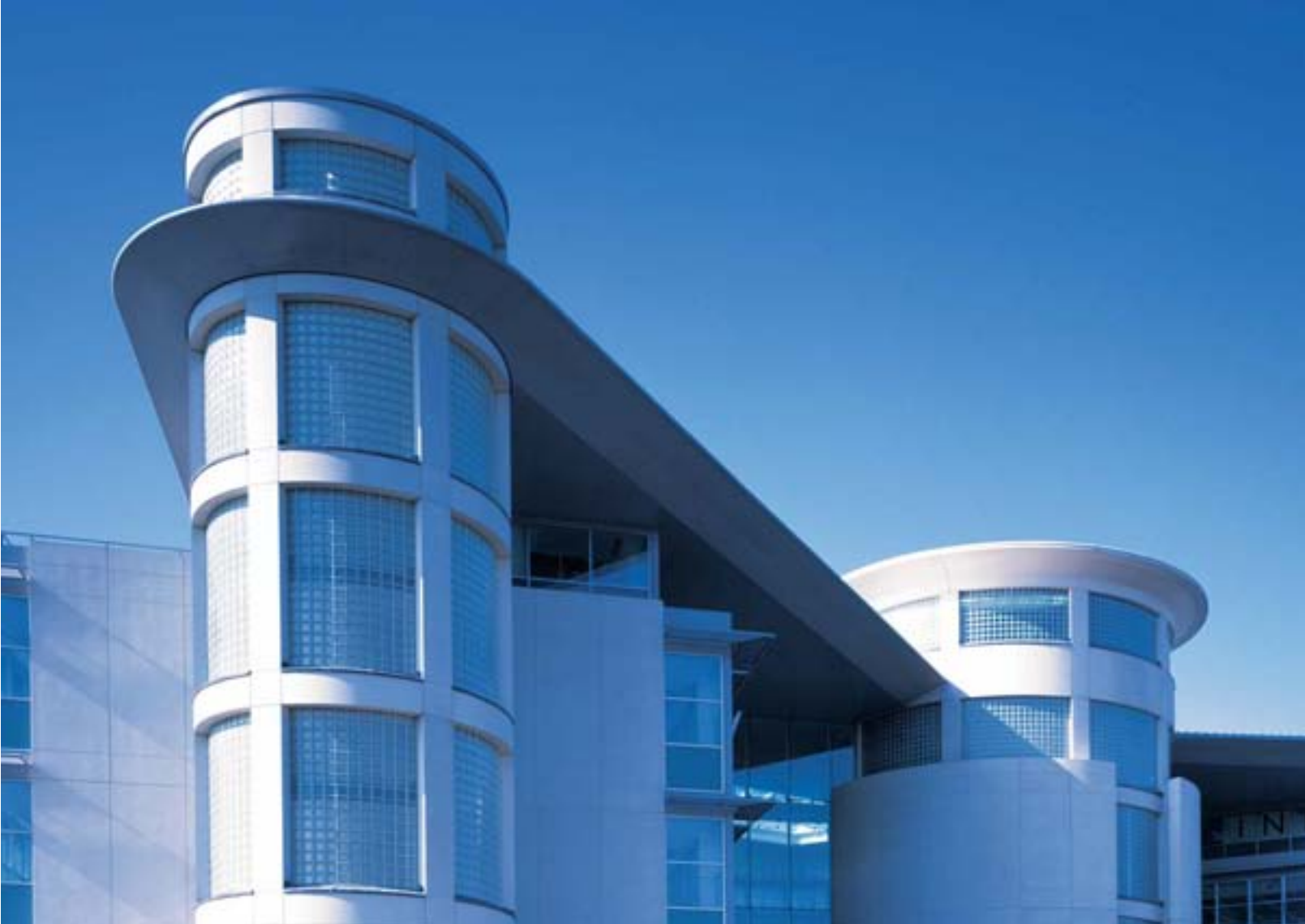
HEADQUARTERS BUILDING, EGHAM
